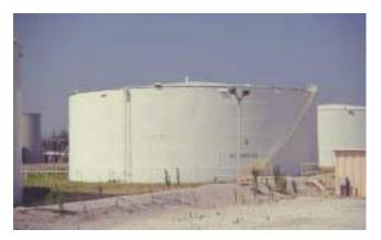
**Figure 25-71** This is a cone roof tank. It has a weak roof-to-shell seam so that in the event of an explosion the roof will come off, but the tank should remain intact.
