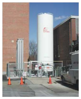
**Figure 25-75** This tank holds cryogenic liquid oxygen and is typical of a cryogenic upright tank.
