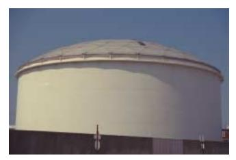
**Figure 25-73** This is a covered floating roof tank, which is the same as an open floating roof tank but has a cover to keep out snow, rain, and debris. Another term for this type of tank is *geodesic domed tank*.
