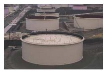
**Figure 25-72** This is an open floating roof tank, in which the roof floats on top of the product. This reduces the release of vapors, as there is no vapor space, and reduces the fire potential.
