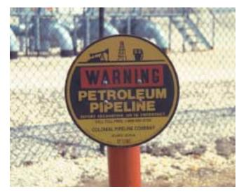
**Figure 25-29** The owner of a pipeline is required to provide the contents of the pipe, the owner's name, and an emergency contact number.
