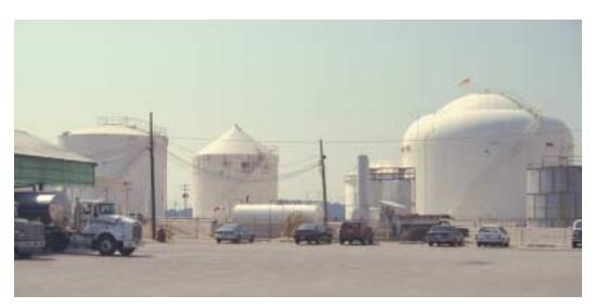
**Figure 25-68** The sizes of tanks vary from a few hundred gallons up to several million gallons. A catastrophic failure of the tank may overwhelm the responders' ability to handle the incident.
