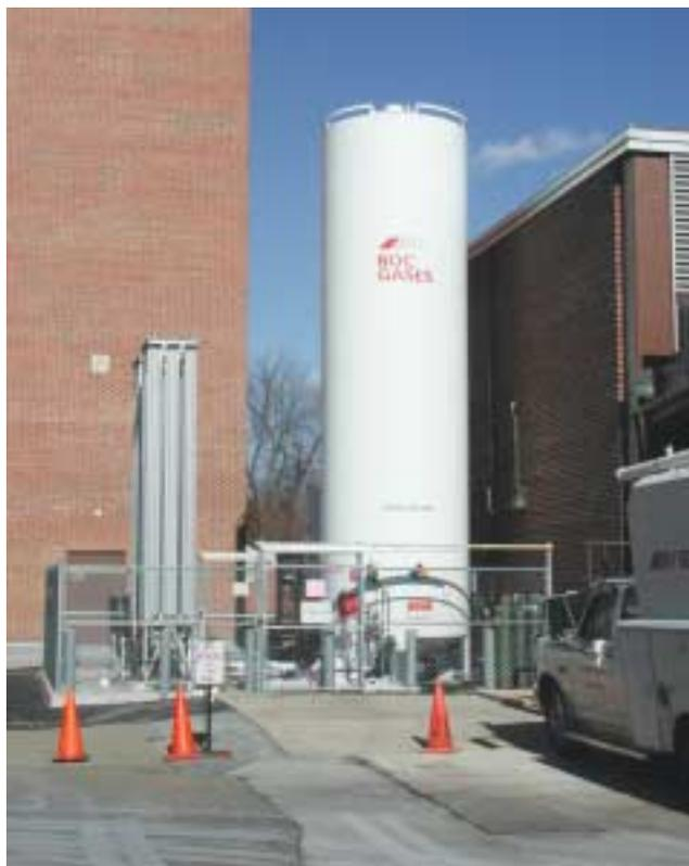
**Figure 25-75** This tank holds cryogenic liquid oxygen and is typical of a cryogenic upright tank.
