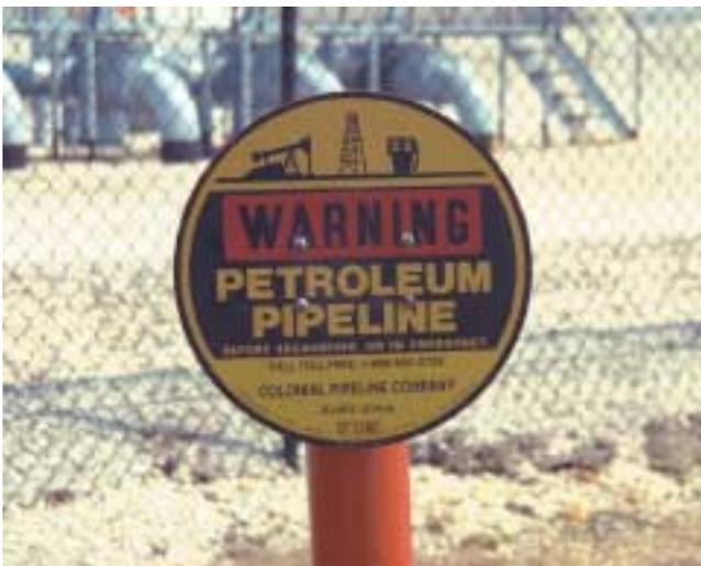
**Figure 25-29** The owner of a pipeline is required to provide the contents of the pipe, the owner's name, and an emergency contact number.
