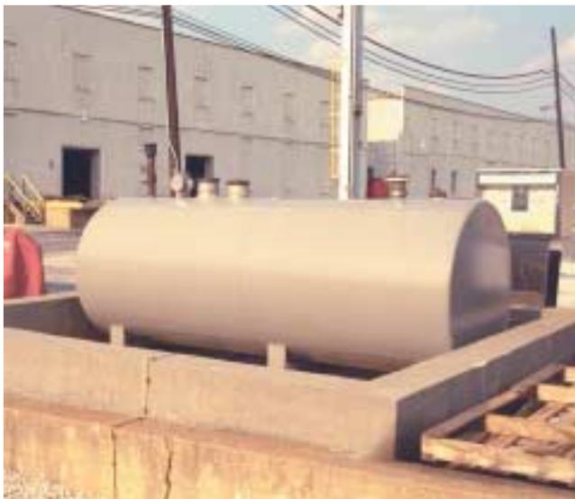
**Figure 25-70** Due to increased environmental concerns, many tanks are being placed aboveground and are called aboveground storage tanks or ASTs.
